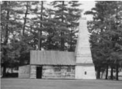
A replica of Drake's second well house and derrick is located on the grounds of the Drake Well Museum in Titusville, Pa. Visitors can enter the wooden building and see the simulated pumping process, which uses a steam engine and a boiler. Drake's drilling tools are on display inside the main museum building.
